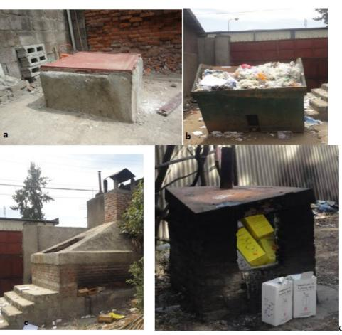
Figure 2 shows the waste disposal system of hospitals (a) placenta pit (b) garbage bin for general waste (c) incinerator for infectious waste and (d) incinerator for needle
