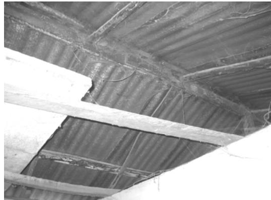
The design of the roofing system as well as the materials used is varied throughout the community. However, hipped and gabled roof types are the basic roof systems used with a pitch of between 20° and 35°. The rafter-purlin system is employed in constructing the roofing structure (Fig. 2b). The roof covering is usually made of corrugated aluminium or asbestos sheets. About 9% of the buildings, mainly of landcrete blocks, have thatch finish (Fig. 3a).
