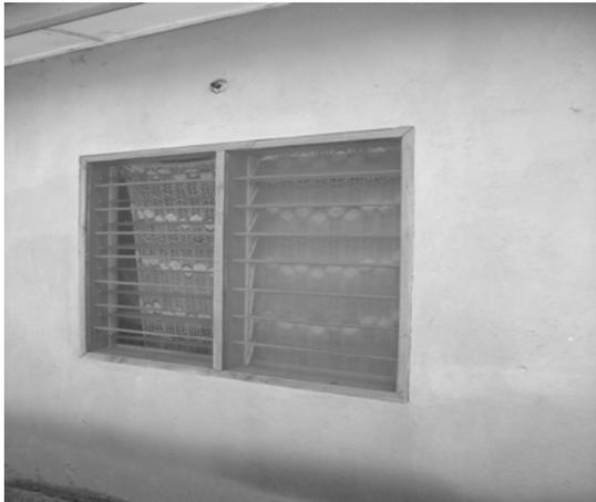
**Fig. 4b: Sun-dried bricks with coating of cement-sand finish in parallel with openings**
