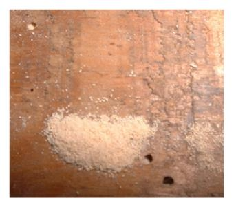
**Figure 1.** Small pile of dust accumulates near exit holes of *A. punctatum* in the wood.
