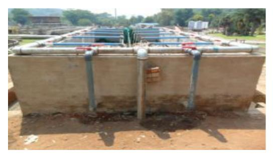
**Figure 3.** Front view of the multi-engineerd system. The middle vertical pipe comes from the tank. The vertical pipes on the left and right are the pipes to the bottom inlet for subsurface flow. Small pipes on top of the bed along the wetland are for vertical flow, while those of surface flow are at the inside front of the system.
