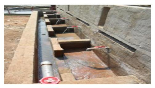
**Figure 4.** Basins and waste channel with a bypass outlet option in the left hand bottom corner of the multi-engineerd system constructed at Kingsburgh, Durban.
