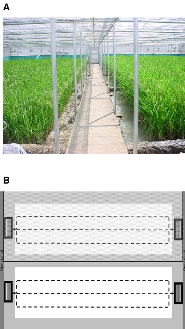
**Figure 2.** Design of screen house for drought screening of GM rice. (A) General view, with a drought-stressed drained plot covered as rainout shelter (left) and flooded well-watered control (right). (B) Each plot is equipped with three drainage pipes (dashed lines) that are connected at each end of the bed to a sump pit.
