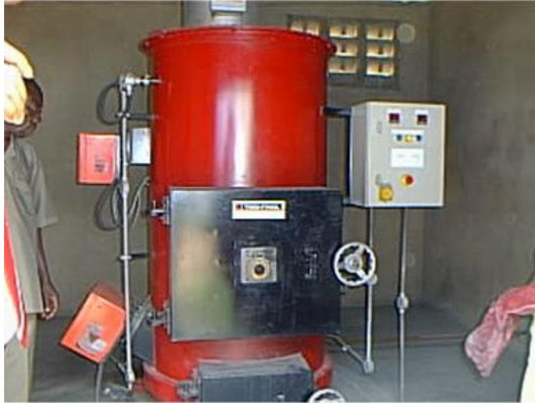
**Plate 4.** Over-utilized incinerator at UCH Ibadan.
