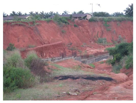
**Plate 1.** Ogbesan Gully, Benin City showing school building caving in and the failed community effort of drain construction to solve the gully problem.
