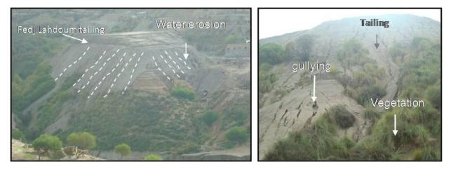
Figure 8. Gullying process in the tailings.
