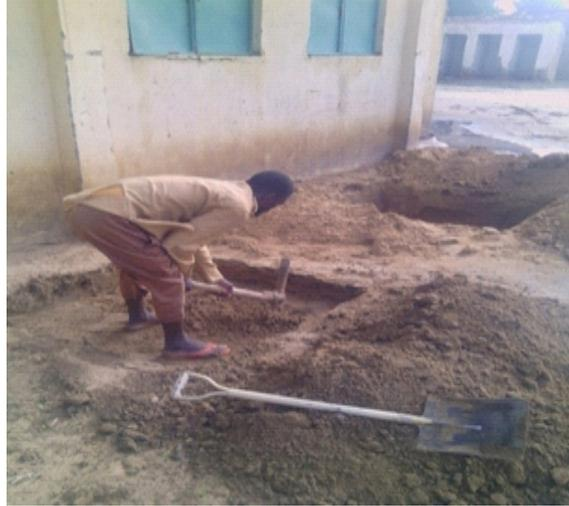
*Plate I: Pits to access the foundation*
