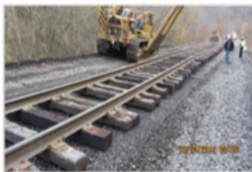
Image 1: Geogrid placement and track restoration (Xiaoqiang and Jiankun, 2019).
