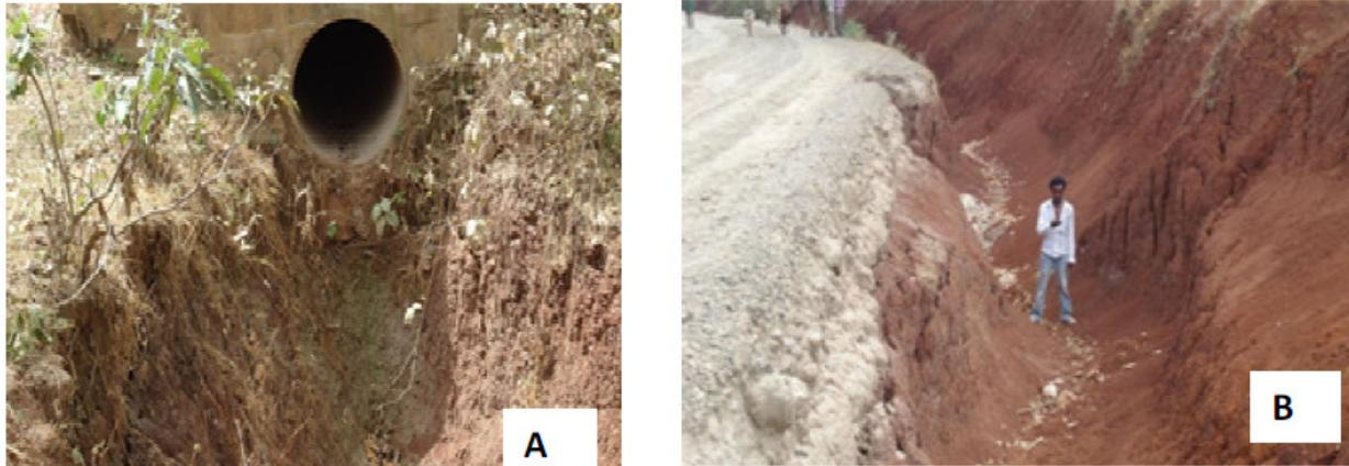
Figure 3: The gully associated with culvert (A) and the gully associated with roadside ditch (B)
