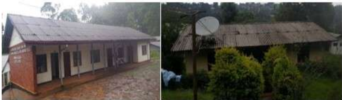
Figure 3: Evangelical Church, Mekane Yesus Central Synod offices, churches, schools, and residence buildings made of AS material in the Nekemete town of western Ethiopia.
