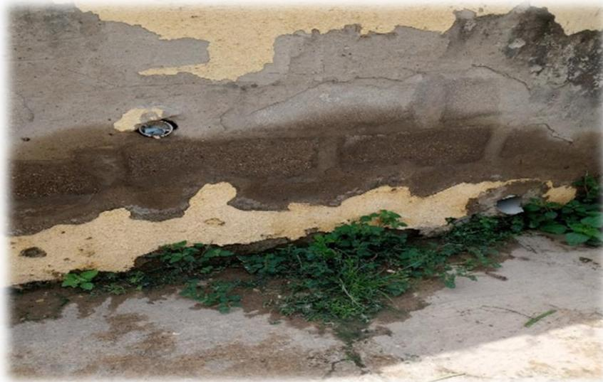
**Figure 2:** Blistering and flaking of mortar within the North Central Region
