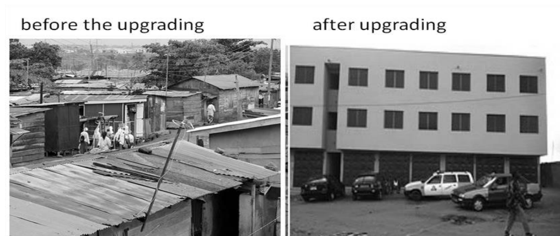
Photo 1 Amui Dzor, before and after upgrading
