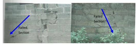
Plate 1: Structural failure as observed on the wall Plate 2: Structural failure as observed on the wall
