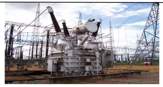
Figure 5: 75MVAR Reactor Located at Benin 330kV Transmission Station
