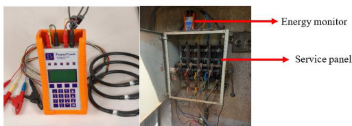
Fig. 3-1: The Power track energy analyser and verifier installed at study site
