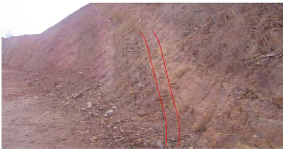
**Fig. 1 Unstable Pitwall showing Tension Cracks (in red) at Initial Excavation Stage**
