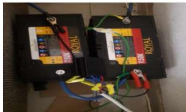
Figure. 3. 2x 12V 100 Ah VRLA Batteries coupled to the Soweto SWT
