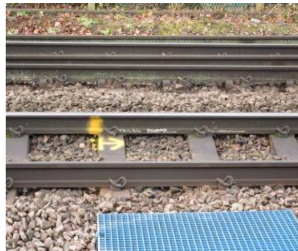
Fig. 1: A Continuously Welded Rail (CWR) Track (Source: Jones and Ashby, 2019).
