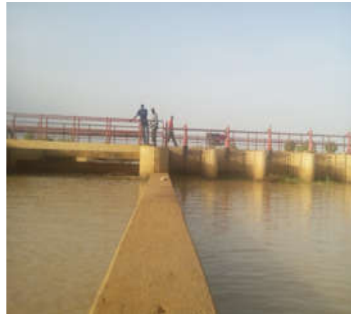
Plate 7: Hadejia Dam Barrage along Hadejia-Nguru wetlands
