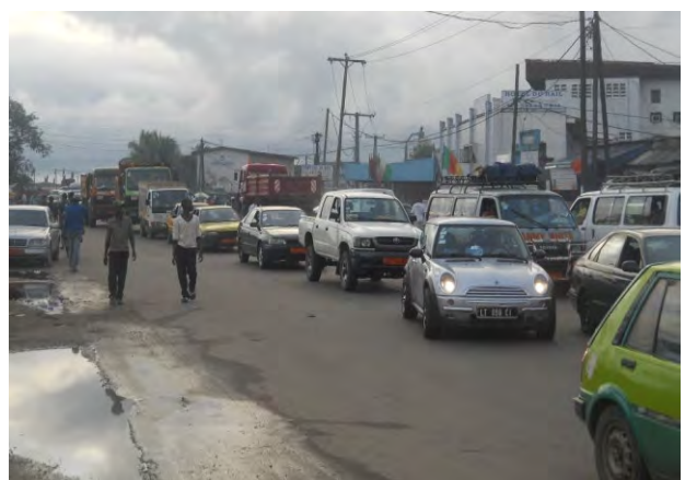
Figure4. 8-10 Potholes and Pre-Congestion conditions at Rail - Bonabéri. Source: Authors' Collections
