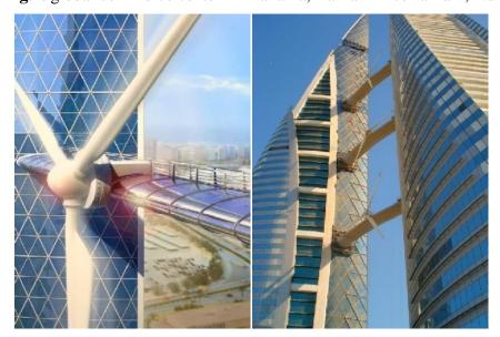
Fig.5. the view of three wind turbines location between two towers
