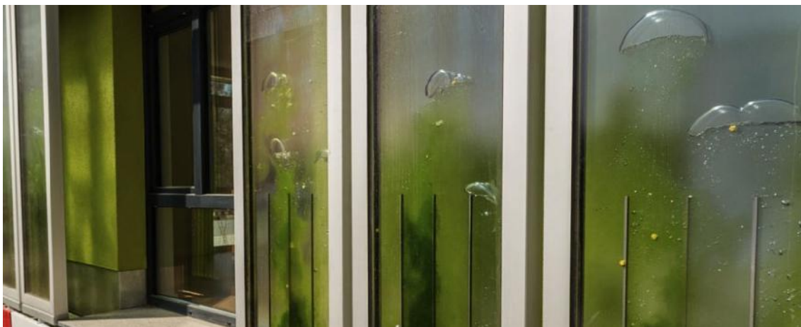
A close view of the Bio-reactors in the building (image 8)
