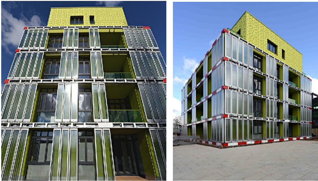
Apr 12, 2013 two sides of the building are clad in panels containing live micro-algae image (9 ,10)
