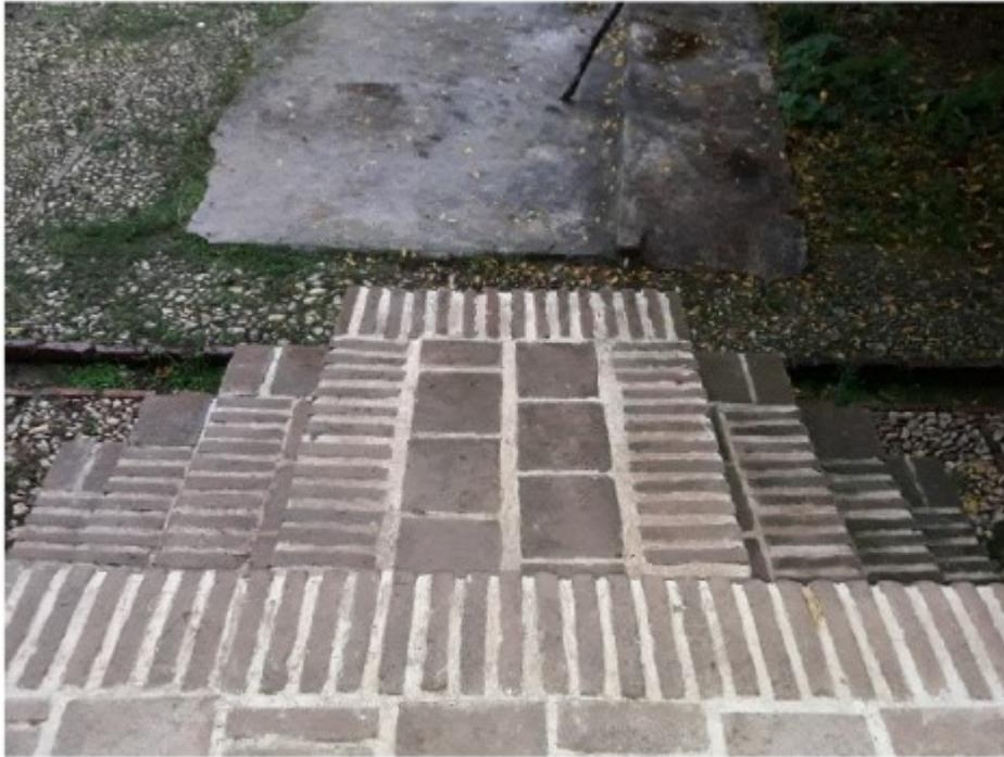
**Fig.7.** Arrangement of bricks for a two-sided stair at entry of the building
