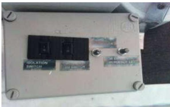
**Fig.21.** Solar circuit and emergency alarm circuit box
