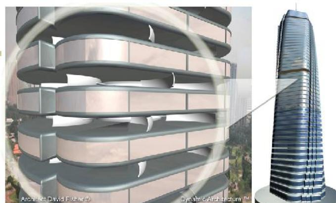
**Fig.7.** the turbine location between floors
