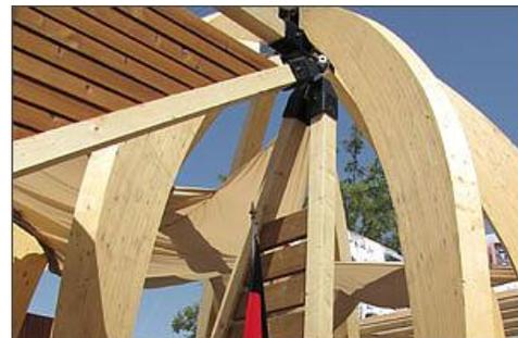
Wooden arches cause less propulsion so they can be readily used over light weight walls. Although, the shape of the arch essentially correlates to the behaviour of the construction
