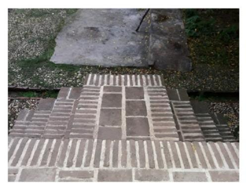
Fig.7. Arrangement of bricks for a two-sided stair at entry of the building
