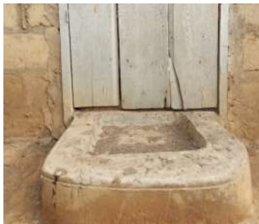
Wrongly sited footbath
