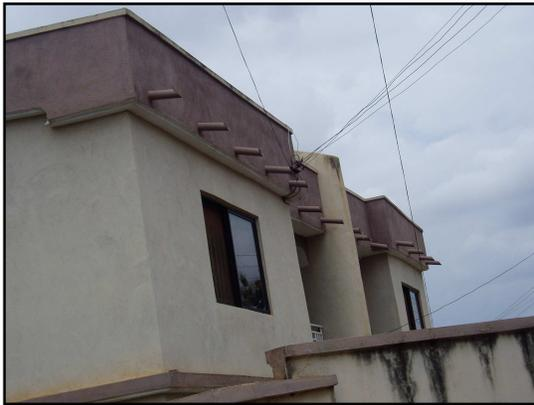
**Plate 6:** Shows the introduction of extra rain water spouts in the parapet walls of the roof to solve the problem of leakage.
