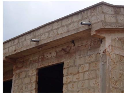
**Plate 3: Example of the use of sandcrete blocks in constructing a parapet wall.**
