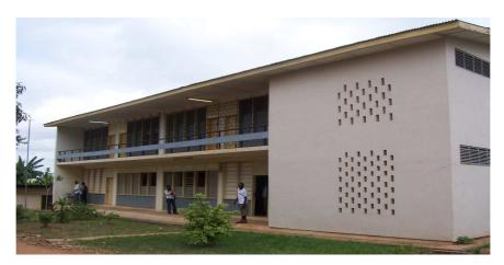
Fig. 3: The Experimental 2-storey Office Block for DHPR on Kwame Nkrumah University Science and Technology (KNUST) campus built with TEK-Block in 1975 (Authors' Field Survey, 2008).
