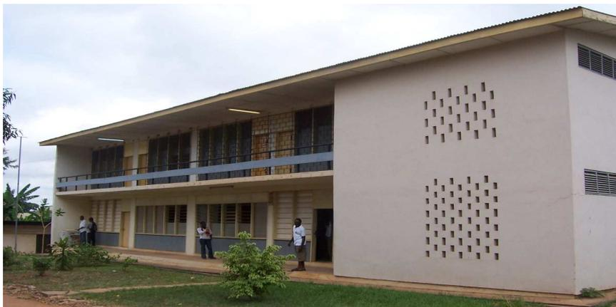
**Fig. 3: The Experimental 2-storey Office Block for DHPR on Kwame Nkrumah University Science and Technology (KNUST) campus built with TEK-Block in 1975** (Authors’ Field Survey, 2008).
