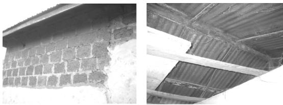
The design of the roofing system as well as the materials used is varied throughout the community. However, hipped and gabled roof types are the basic roof systems used with a pitch of between 20° and 35°. The rafter-purlin system is employed in constructing the roofing structure (Fig. 2b). The roof covering is usually made of corrugated aluminium or asbestos sheets. About 9% of the buildings, mainly of landcrete blocks, have thatch finish (Fig. 3a).
