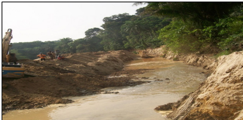
Fig. 6. One of the newly created diversionary paths on the Ankobra River, to allow for gold prospecting on the river bed (Photo: Author)
