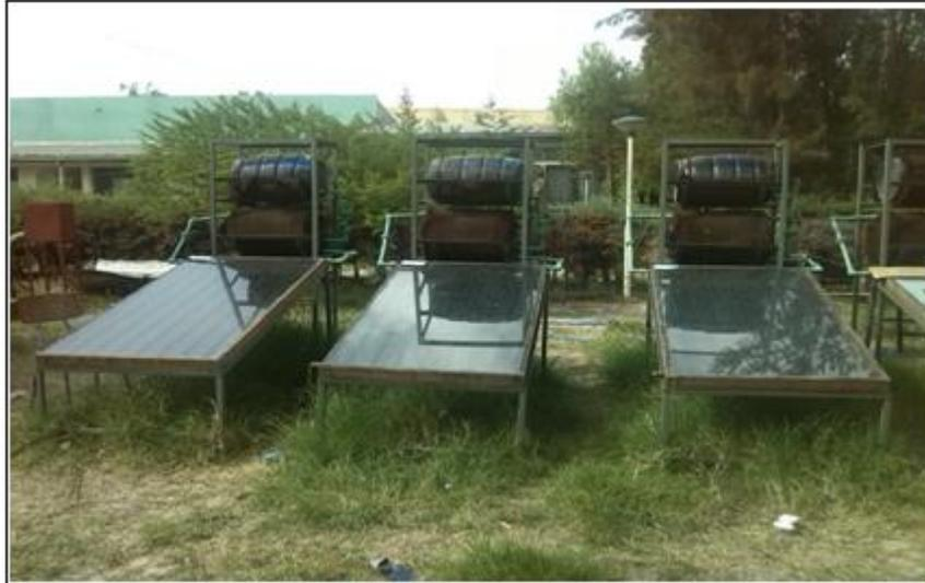
Figure 2. Flat plate solar water heaters.
