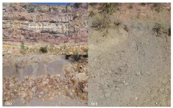
Figure 3. (a) Jointed sandstone unit exposed about 100 m away from the failure section located north west of the study area (b) highly weathered sandstone unit at the contact of the asphalt road failure (c) unconsolidated shale unit exposed along the slide section of the road.
