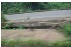
Plate 23. A bridge with collapsed protective handrails along Benin – Lagos Express Way Source: author's field work
