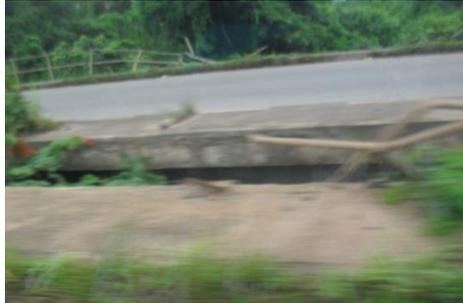
Plate 23. A bridge with collapsed protective handrails along Benin – Lagos Express Way
