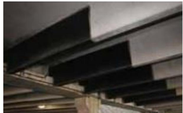
Plate 1: FRP Strengthened reinforced concrete beam [17]
