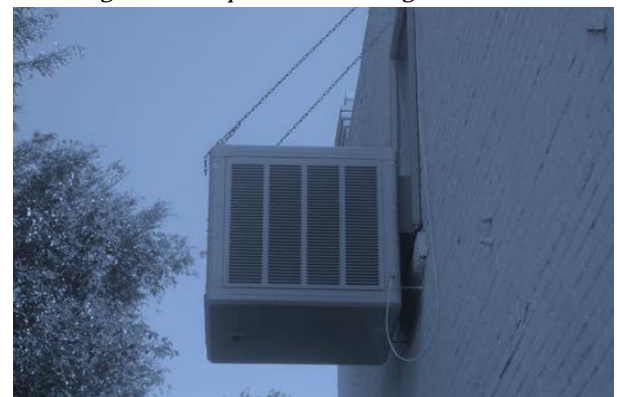
Figure 3: DEC Window Installation
