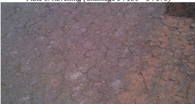
Plate 10: Hair Cracks (Chainage 2+950 - 3+050)
