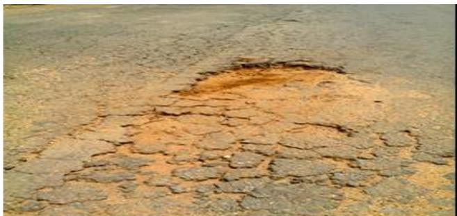
Plate 7: Crocodile Crack and Pothole (Chainage 3+150 - 3+175)
