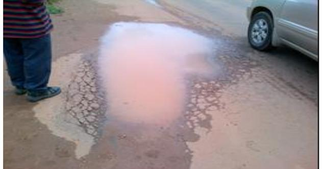
Plate 6: Rut, depression, Cracks, Shoving (Chainage 2+950 - 3+050)
