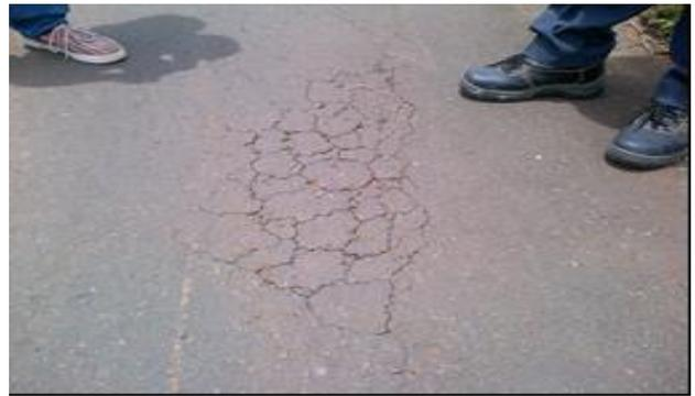
Plate 2: Crocodile Crack (Chainage 2+850 - 2+950)
