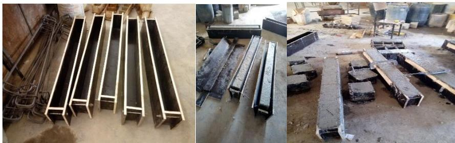
Figure 3: Wooden Formwork, Cast Beams and Cubes
