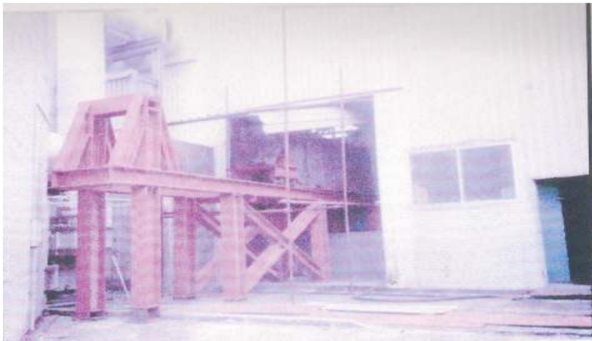
Figure 9: As-built photo of the shaft-sleeve puller mechanism.
