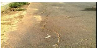
Plate 4: Longitudinal Crack (Chainage 3+050 – 3+100)
