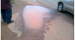
Plate 6: Rut, depression, Cracks, Shoving (Chainage 2+950 – 3+050)
