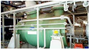
Figure 1: Typical 2BCL Barrel Centrifugal compressor [4]
