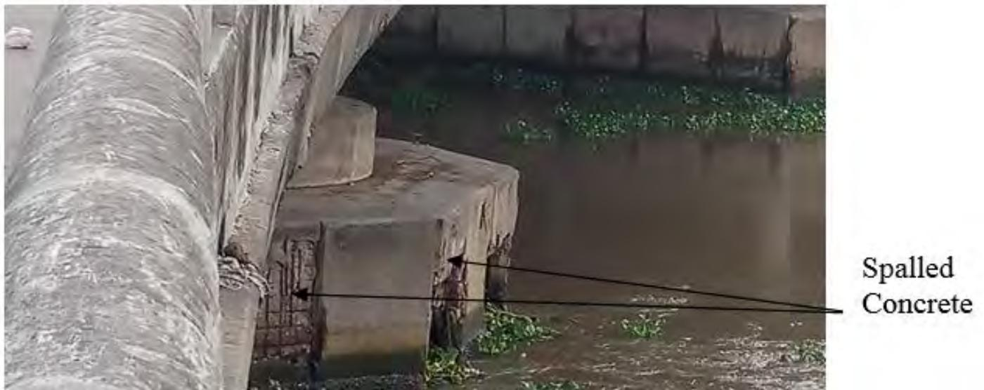
Figure 1: Concrete spalling of the pile cap of Carter bridge in Lagos, Nigeria.
