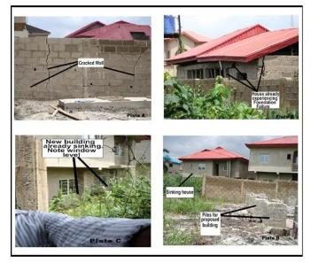
Figure 2: Photographs of cracks that appeared in wall and building at the site (top), and the sinking buildings near the site (bottom).
