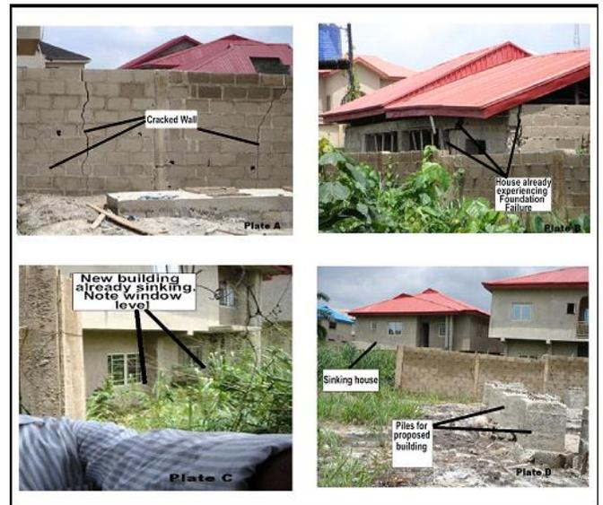
Figure 2: Photographs of cracks that appeared in wall and building at the site (top), and the sinking buildings near the site (bottom).
