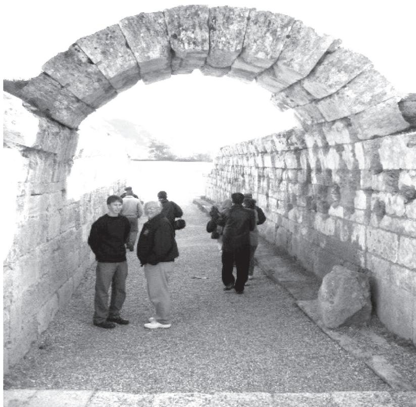
You will note that arches are designed with an odd number of stones, with the top, middle stone being the *keystone* on which the bridge's weight rests. In this case, the top of the arch consists of 11 stones in total, five on each side and the keystone in the middle. These stones have slanted sides so that they fit tight against each other. The downward force of the bridge's weight spreads out to the stones on either side of the keystone through the force of gravity.
